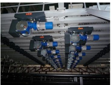
Heavy Duty Lighting Hoist with up to 18 m (59') long traveling connector strip / lighting bar assembly for up to 48 lighting circuits.
